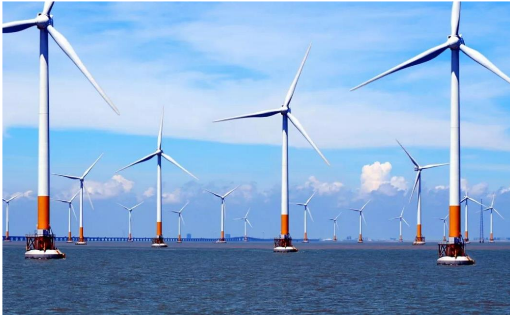
Fig.7. The Offshore Wind Farm in Asia—Shanghai Donghai Bridge Offshore Wind Farm
